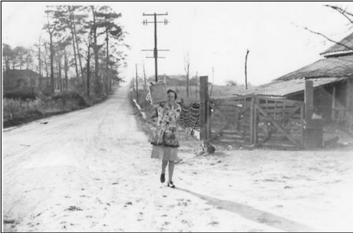
Lula Mae Tyre walking east on unpaved Federal Road from her house to the Pintlala intersection. Note: Grange Hall and Pintlala School, left background, current Mosley's Store location right foreground.
